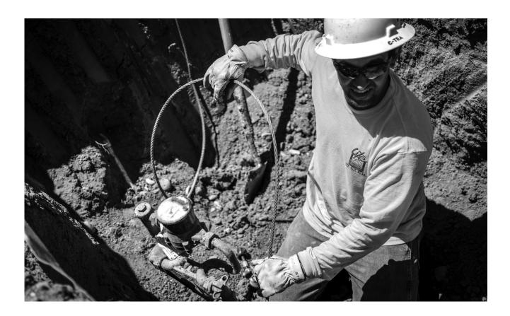
**Above Photo by 14K Media** - Shaun Herrera, Utility Maintenance Worker, runs a cable into a leaking waterline in preparation to replace the line.
