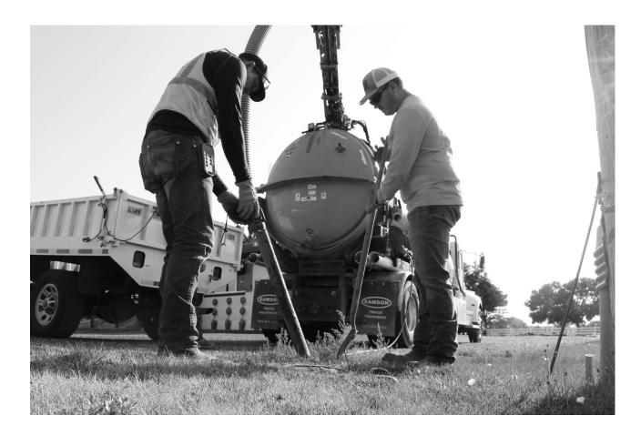
**Above Photo by Andrea Lopez -** Adam Gentzler (left), Utility Maintenance Worker, and Joe Isley (right), Utility Maintenance Worker, inspect a service line for material type using a vacuum truck.
